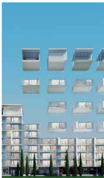
Foto: © CSQUARE/International, csquaremodular.com
